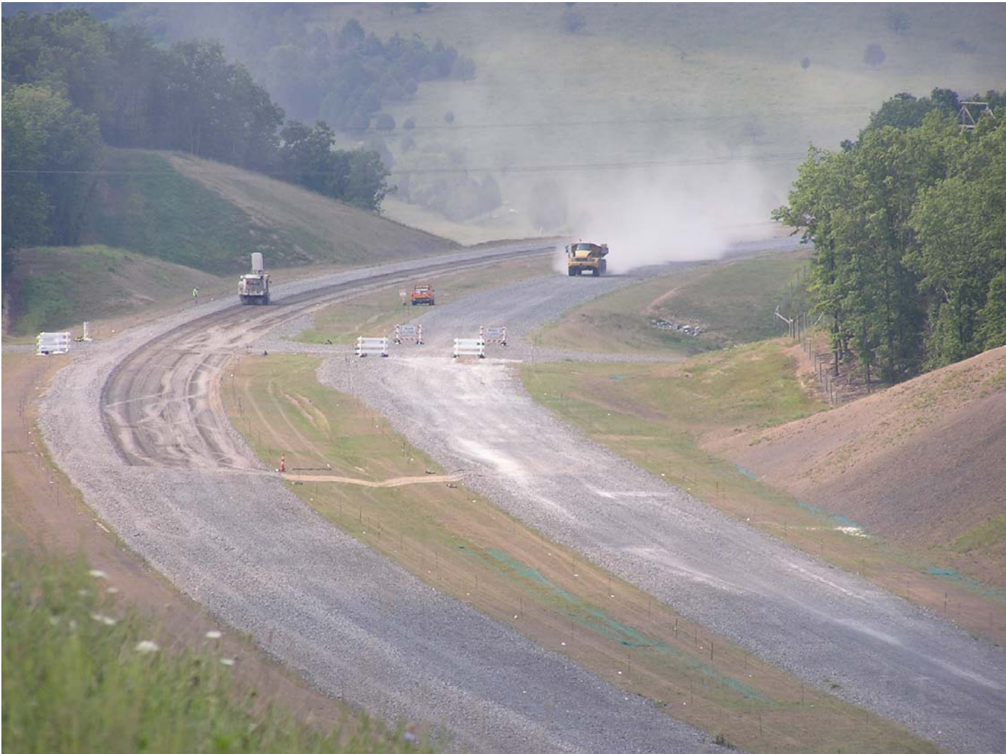
Corridor H – Progress Continues
